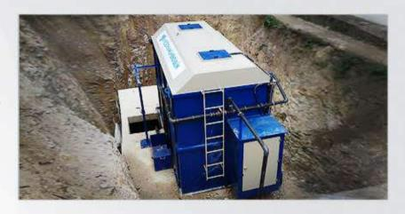
it is an all-in-one wastewater treatment plant for sewage treatment. All of the system running by PLC panel without a labor force.
